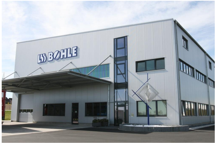
Figure 5 Plant 3 in Ennigerloh
